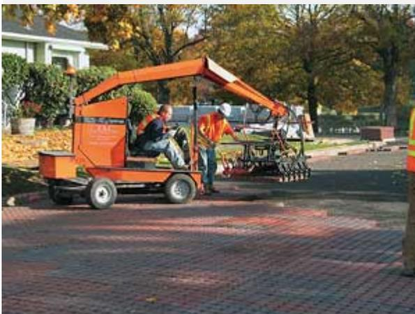
Bob Lisi of LHB Inc. in Duluth, Minn., observes, “The trend is borderline revolutionary in the construction industry. Current pavement design relies on preventing moisture from penetrating the pavement. Porous pavements flip this design practice and readily accommodate moisture in the base materials. My guess is that porous pavements will become mainstream technology across the United States in the next 10 years.”
